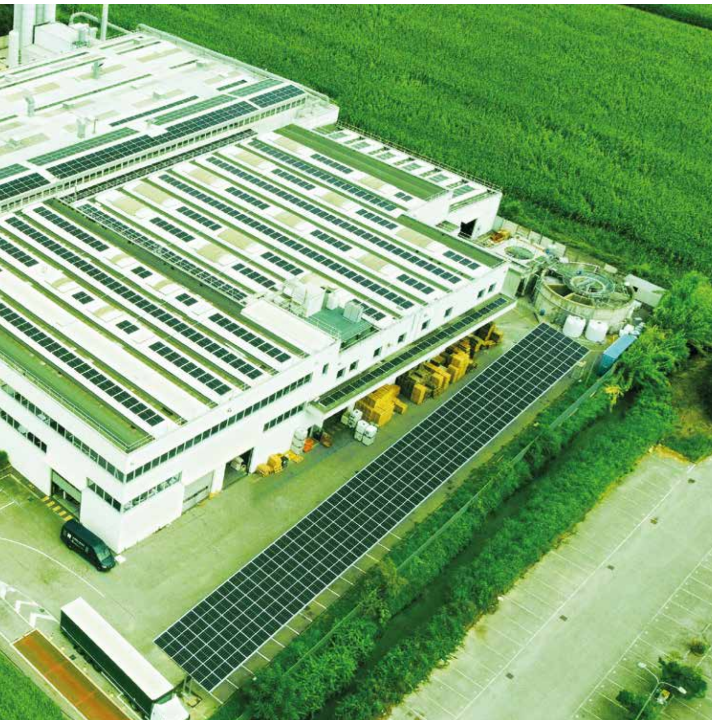
Aerial photography JV spa | November 2024
